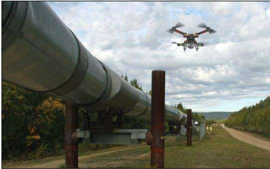
Figure 2.3: Drone Inspection of the Pipeline [58].
