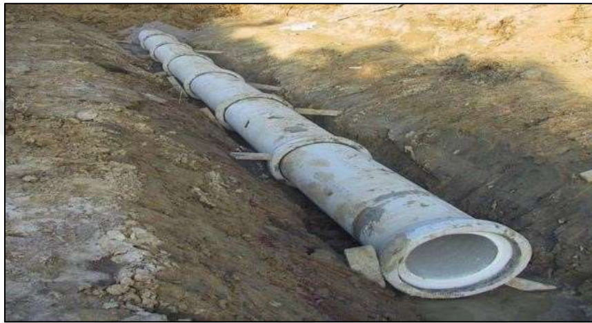
Figure 3.5: The Reinforced Concrete Pipe with a Sheet Metal Core.
