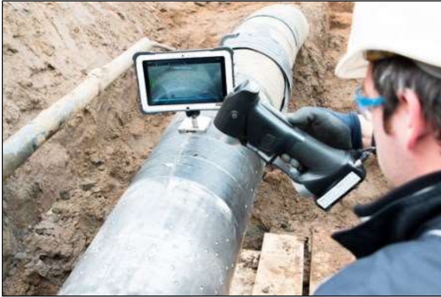
Figure 2.1: Visual Inspection of the Pipeline [45].
