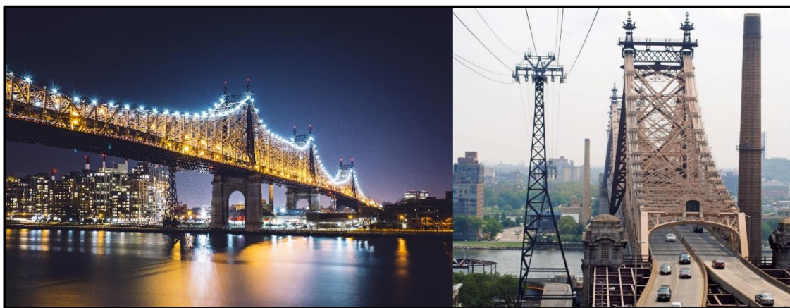
Figure 5.26. The Queensboro Bridge at night (left), the bridge during day time [131].
