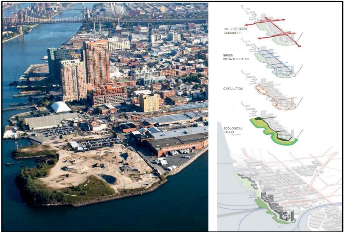
Figure 5.14. Hunter's Point South Park design process along with the ongoing construction photograph [137].
