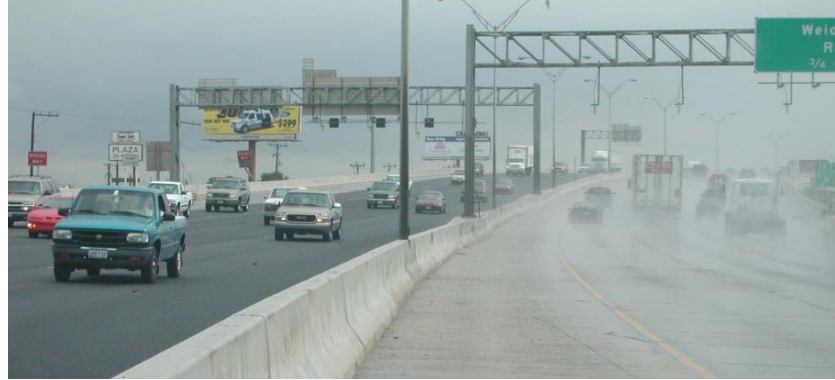
Figure 3.3 Visibility of permeable asphalt and conventional asphalt pavements in rainy weather (Topaloglu, 2019)
