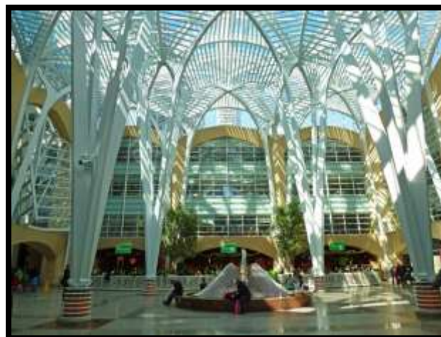
Figure 2.21: The Ceiling Structure in Toronto (RedPat, 2014).
