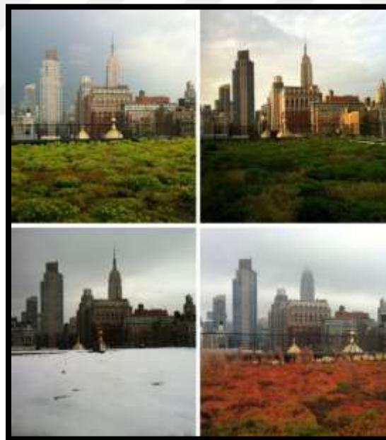
Figure 2.18: The Greenroof of COOKFOX Architects' New York (Browning et al.,
