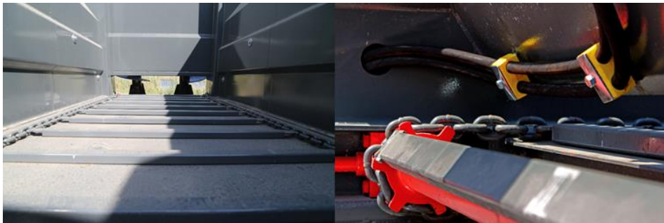
Figure 3.4. Conveyor mechanism inside trailer
