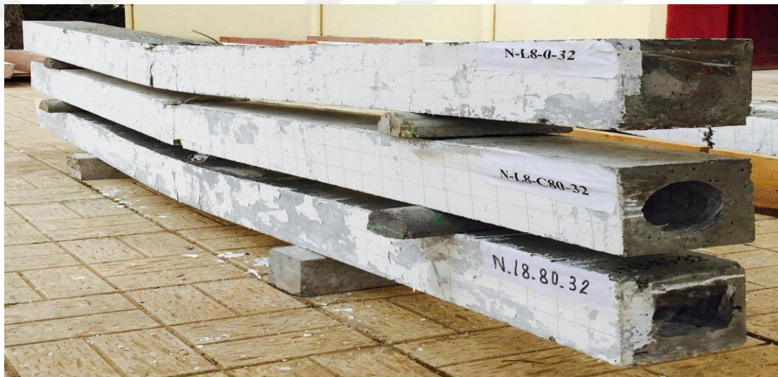
Figure 4.20 Structural failure for beam specimens of Group B.
