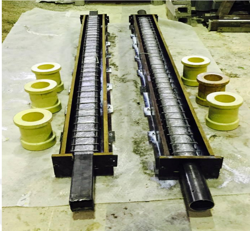
Figure 3.8 Fabrication process of hollow specimens with stirrups.
