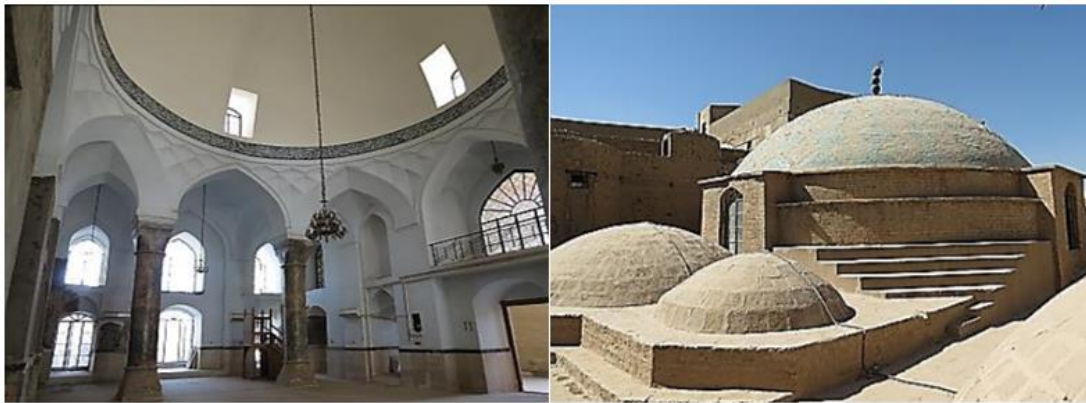
Figure 4.10. The dome of Al-Mouradia Mosque and the columns supporting it from the inside and outside (Fahmi, 2018, p. 13).
