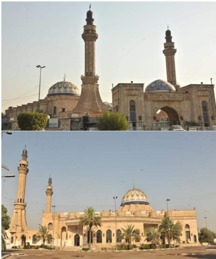
Figure 4.19. The front and side of Al-Nida Mosque (Photograph taken by author)
