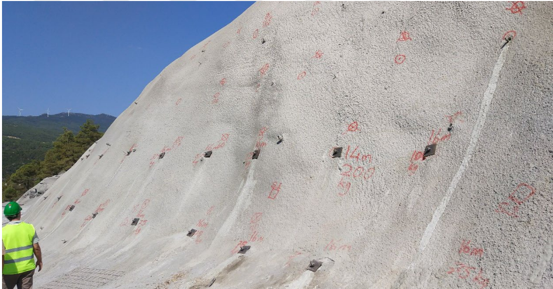
Figure 3.15 The application of the shotcrete and rock bolts on the bench surface (Personal archive, 2019)
