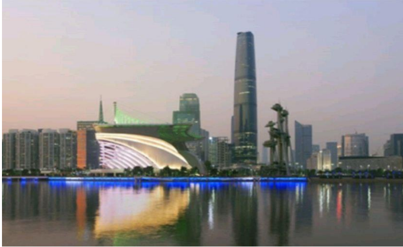
Figure 3.1. Guangzhou Opera House, its distinctive pebble shape can be seen on the banks of the river (Sebastian et al., 2018).
