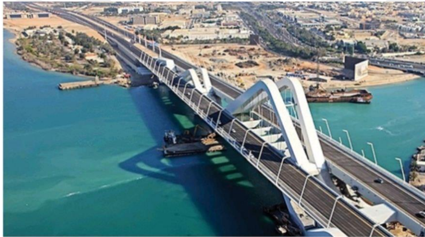
Figure 3.17. Sheikh Zayed Bridge, the bridge's distinctive luminance and spine can be seen (Nisreen, 2020).
