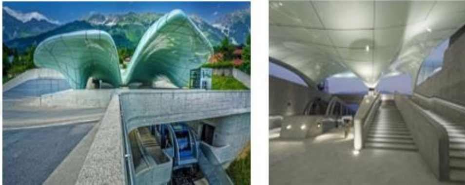
Figure 3.13. Nordpark Railway Stations, formal curves in the external surfaces as complementary elements to the formation structure (Abdalwahid, 2013).
