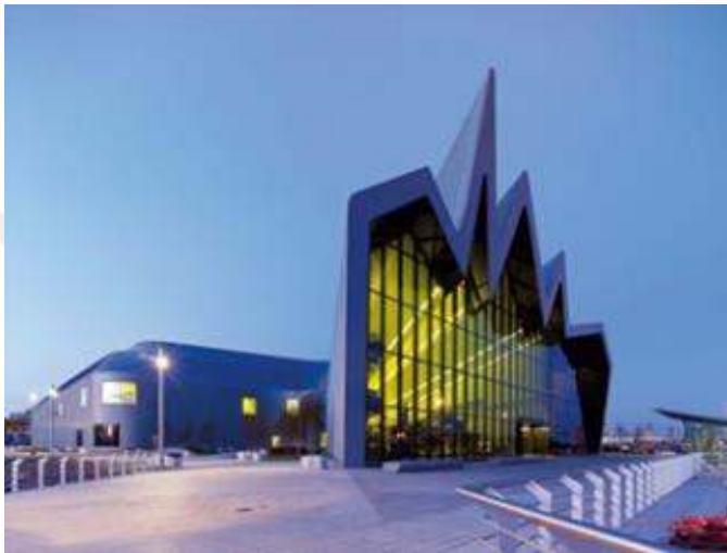
Figure 3.21. The exterior design of Riverside Museum Architects (Sebastian et al., 2018).
