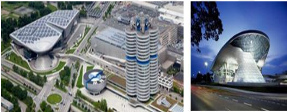
Figure 3.6. Flying roofs in the BMW building (Sebastian et al., 2018).
