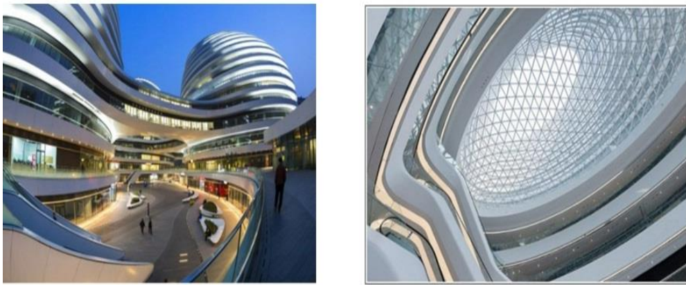
Figure 3.15. Galaxy SOHO, the interior is covered with glass, while the outer surface is covered with aluminum and stone, 2009-2012, China (Youns, 2017).
