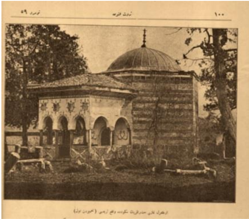
Fig. 32 “His Royal Highness Ertuğrul Gazi’s Mausoleum situated in Söğüt (before repairs)”, Ahmet Ersoy, “The Sultan and His Tribe” 45, fig. 10.
