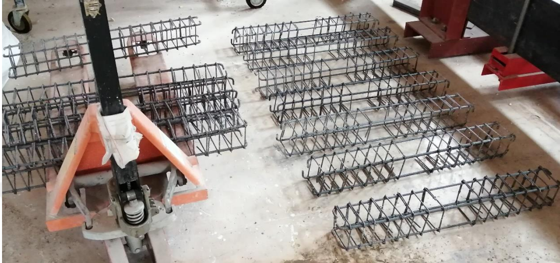
Figure 3.2 Beams reinforcement cages
