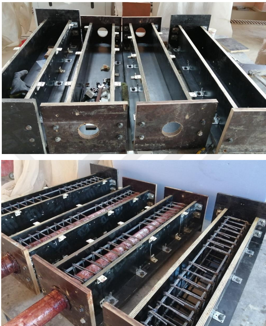
Figure 3.3 Details of beams molds
