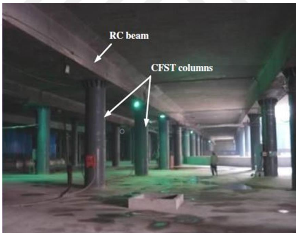
Figure 1.2 Subway station in Tianjin(Han and Bjorhovde, 2014).
