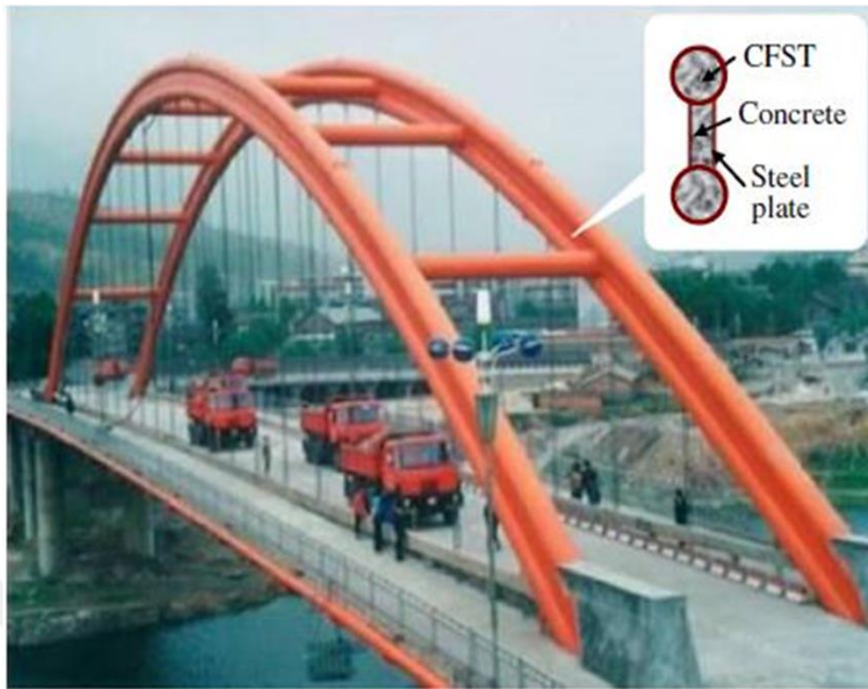
Figure 1.1 Wangcang East river bridge (Han and Bjorhovde, 2014).
