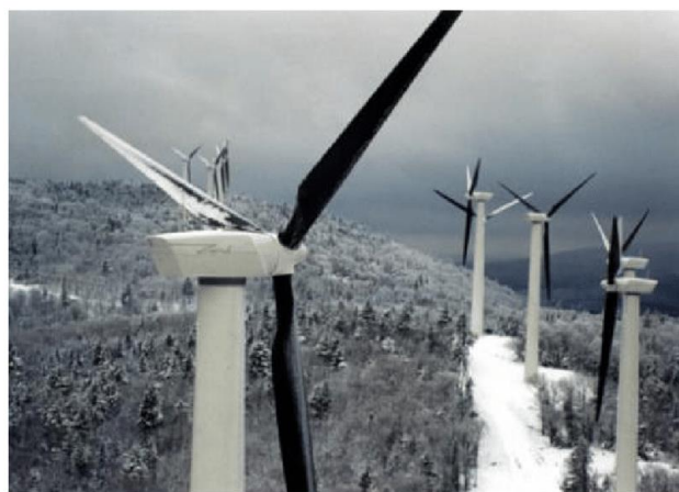
Figure 13. Black paint on the blades of HAWT [26]
