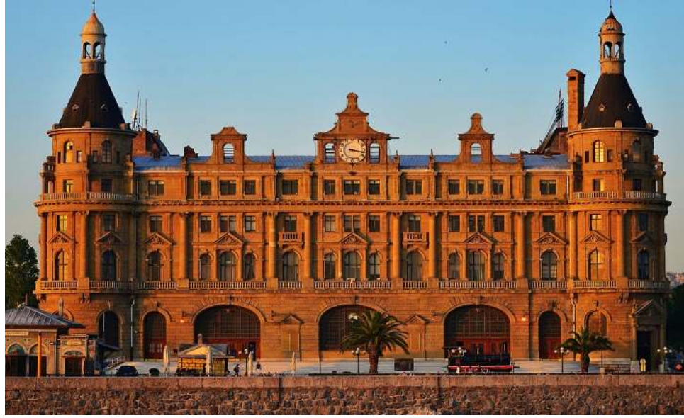
Figure 57: Haydarpaşa Train Station Facade (URL50)
