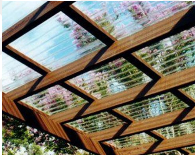
Figure 6.35 Photo illustrating PVC roofing implementation [175]
