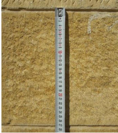
Figure 6.4 Photo of the Topaktaş stone in Gaziantep railway station [76]
