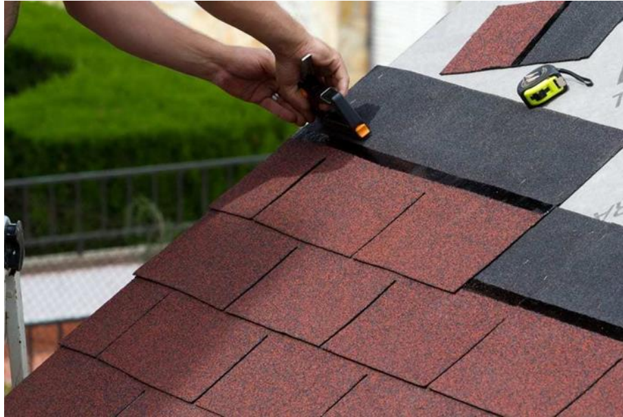
Figure 6.32 Photo of an asphalt shingle implementation
