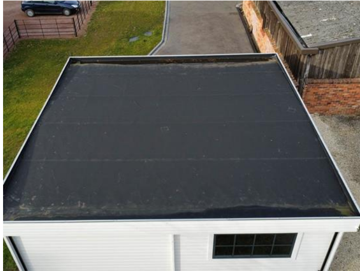
Figure 6.33 Photo of roofing membrane implementation [173]
