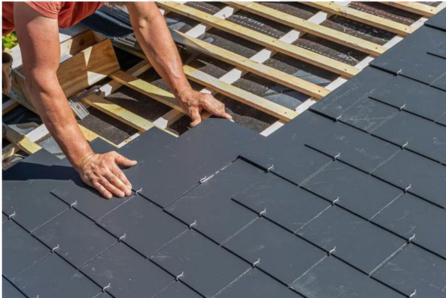
Figure 6.41 Photo illustrating slate roofing implementation [182]
