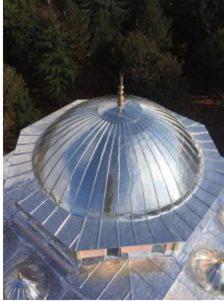
Figure 6.25 Flat aluminum sheet implementation on the dome of a mosque [162]
