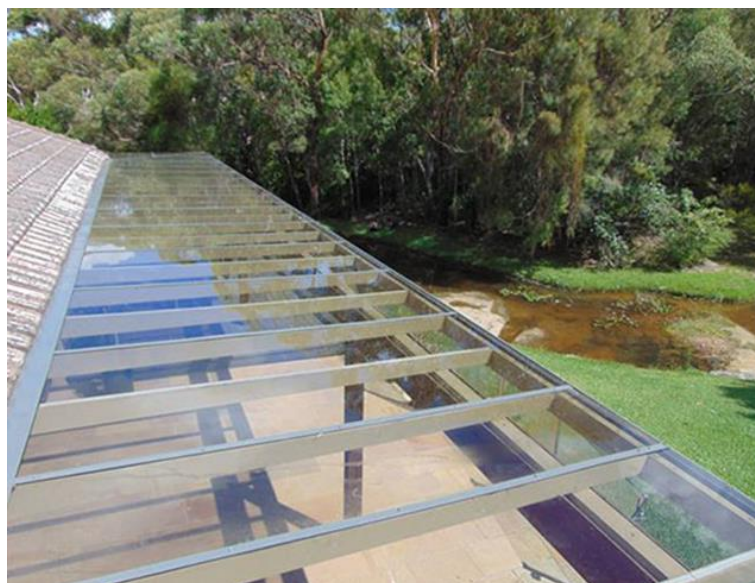
Figure 6.37 Photo illustrating acrylic glass roofing implementation [177]
