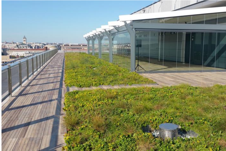
Figure 6.42 Photo illustrating planted roofing [183]
