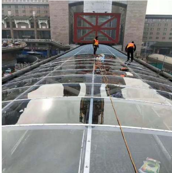
Figure 6.36 Photo illustrating polycarbonate roofing implementation [176]
