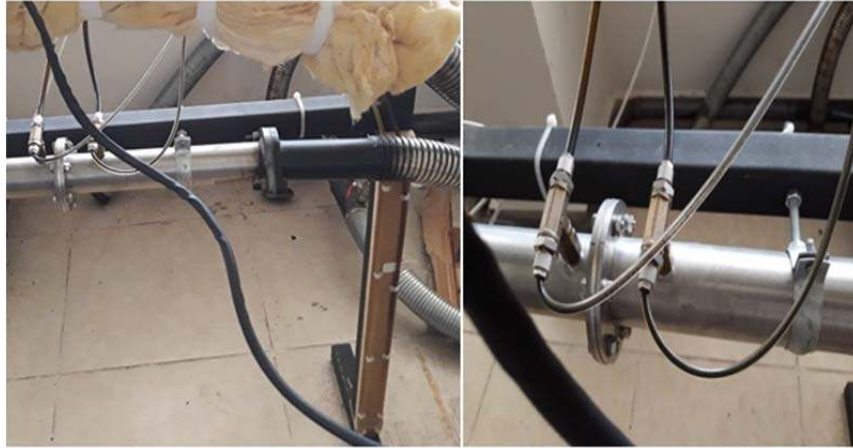
Figure 5.16. Manometer with an orifice plate
