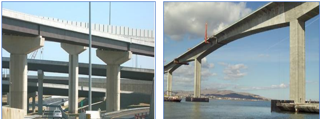
Figure 1.1 Reinforced Concrete Haunched Beams (RCHBs)
