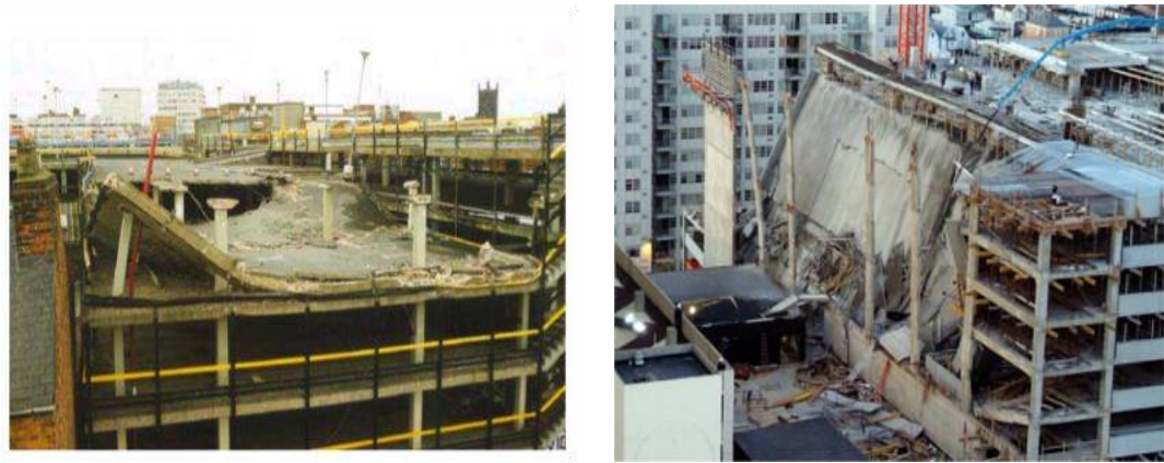
Figure 1.1 An example of punching shear.
