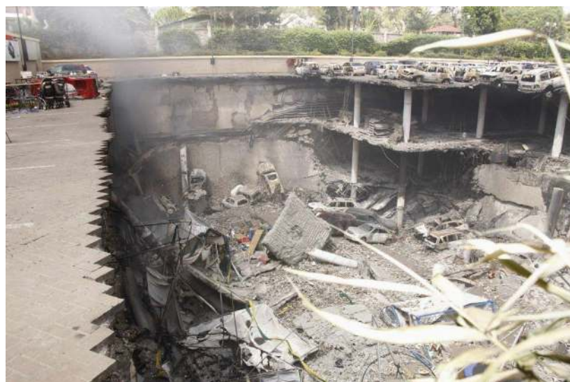
Figure 1.2 Building collapsing due to fire (Westgate mall)
