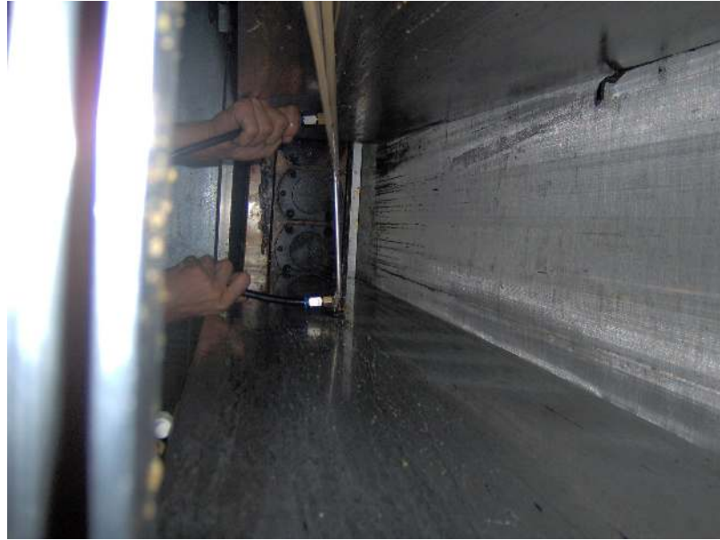
Figure 4.15 Adjusted the cooling pipe by hand.
