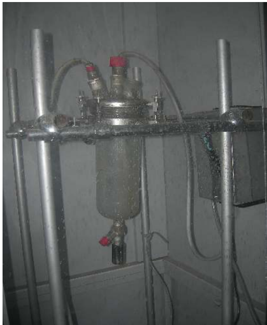
Figure 3.2 View of ozone treatment system
