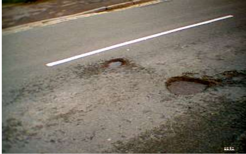
Figure 1.3: Crack in the Road.
