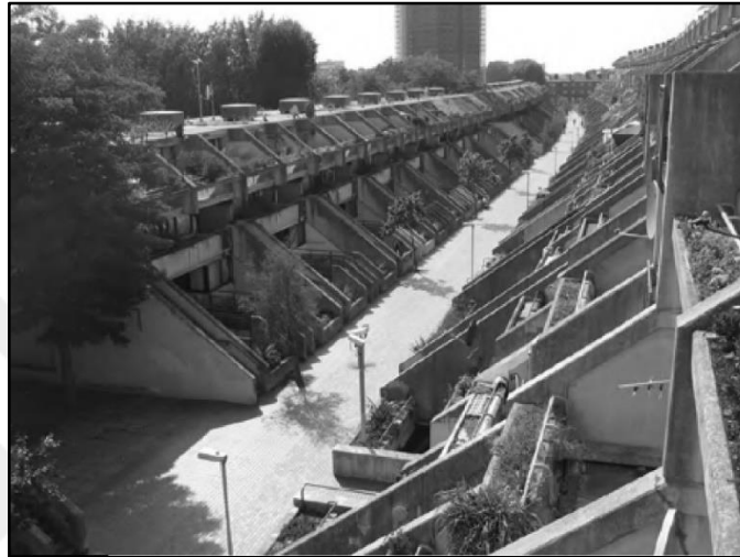
Figure 2.6. Neave Brown, Alexandra Road Estate [8].
