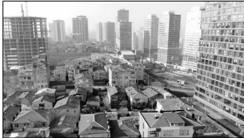
Figure 3.17. Fikirtepe regeneration project area [58].
