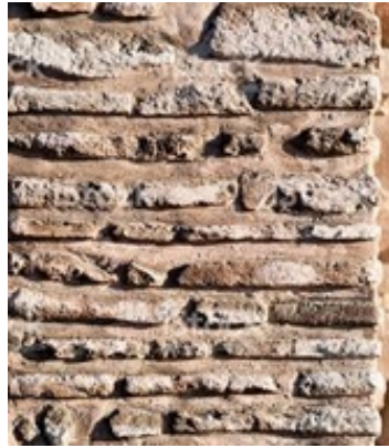
Figure 2.4. The mortar layer between the bricks [18].
