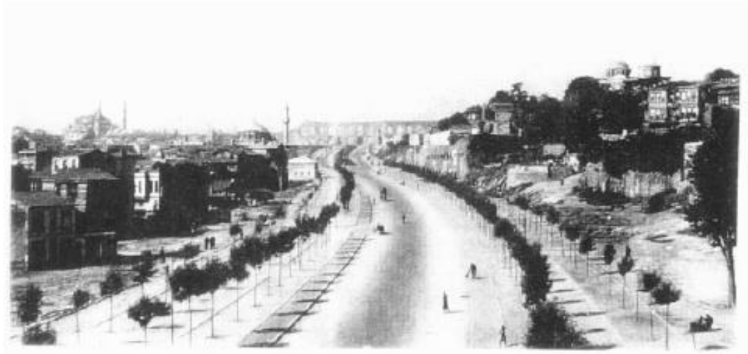
Figure 3.5 Atatürk Boulevard, Symbol of the Road-Making Agenda in the Context of Urban Voids
