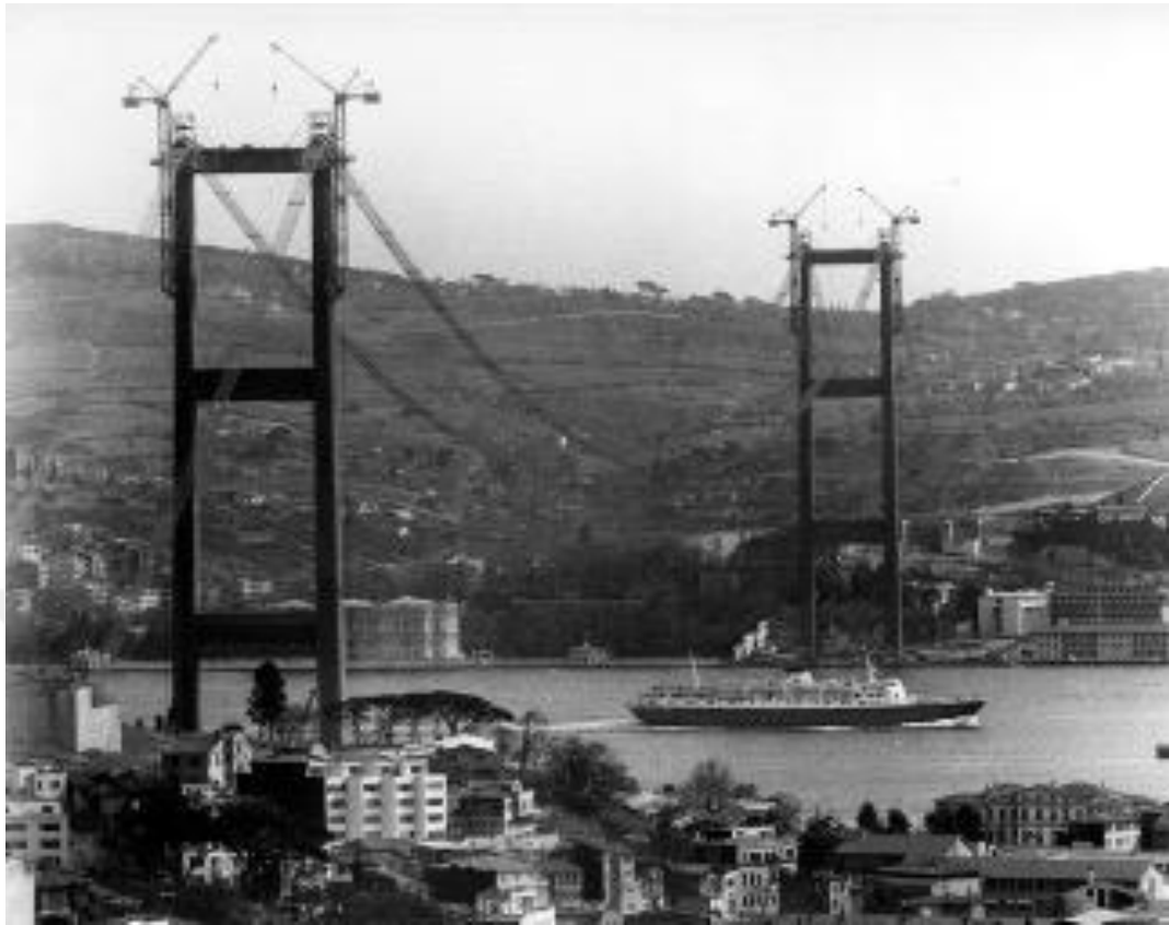
Figure 4.4 First Bridge over the Bosphorus. Yapı Kredi Archive.
