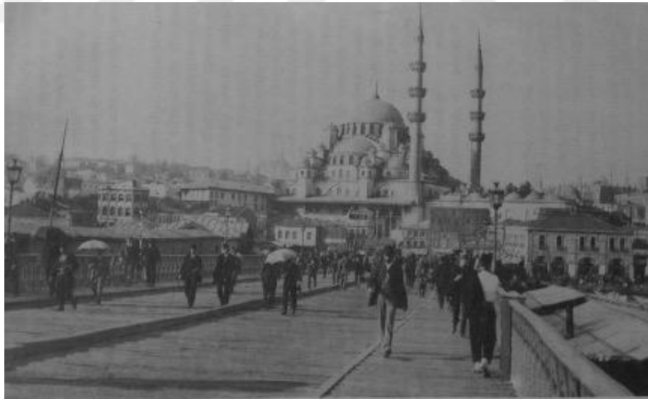
Figure 2.9 "Third Galata Bridge, 1878, which had iron construction and wooden pavements hard to walk on for strangers." Hagop Mintzuri. İstanbul Anıları 1897- 1940 , Tarih Vakfı Yurt Yayınları, 152. 3. Baskı, 1998.
