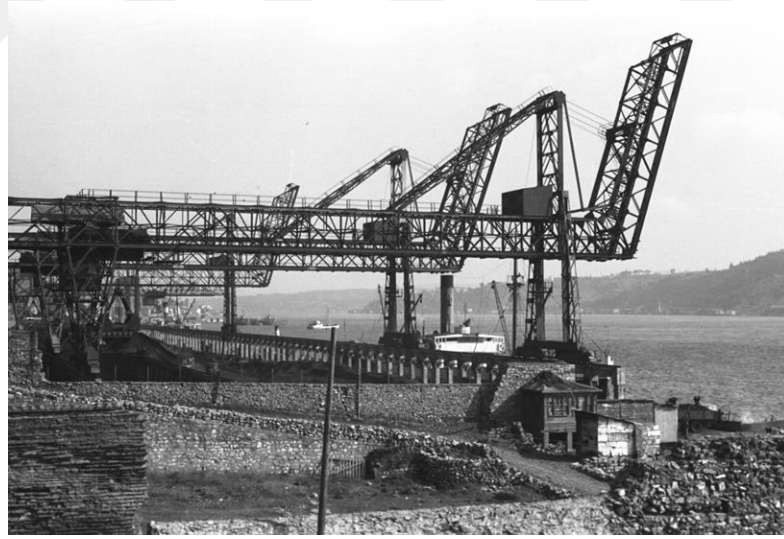
Figure 4.17 The Coal Plant of Kuruçeşme. Högg, 1959 Alman Arkeoloji Enstiüsü, D-DAI-IST-KB 11.443
