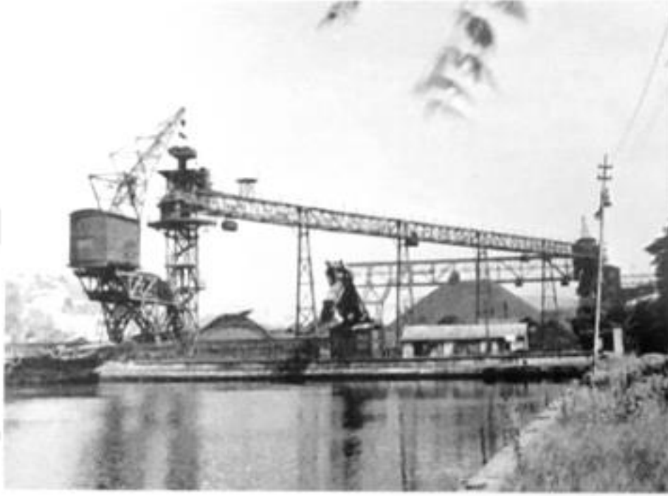
Figure 4.20 Dock Crane, Barge, Coal Park, and Overhead Line of Silahtarğa Power Plant in 1970. TEDAŞ Photo Film Center Archive in Asu Aksoy (edt) Silahtarğa Elektrik Santrali 1910-2004. İstanbul Bilgi Üniversitesi Yayınları, 38, 2007.
