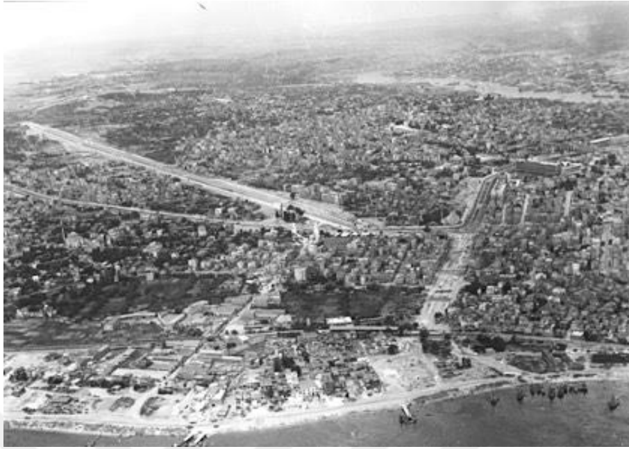
Figure 4.9 During the Construction of Vatan Boulevard, Three Thousand Trees Were Cut Down. Hilmi Şahenk, 1960. Alman Arkeoloji Enstitüsü, D-DAI-IST-R 32.782.
