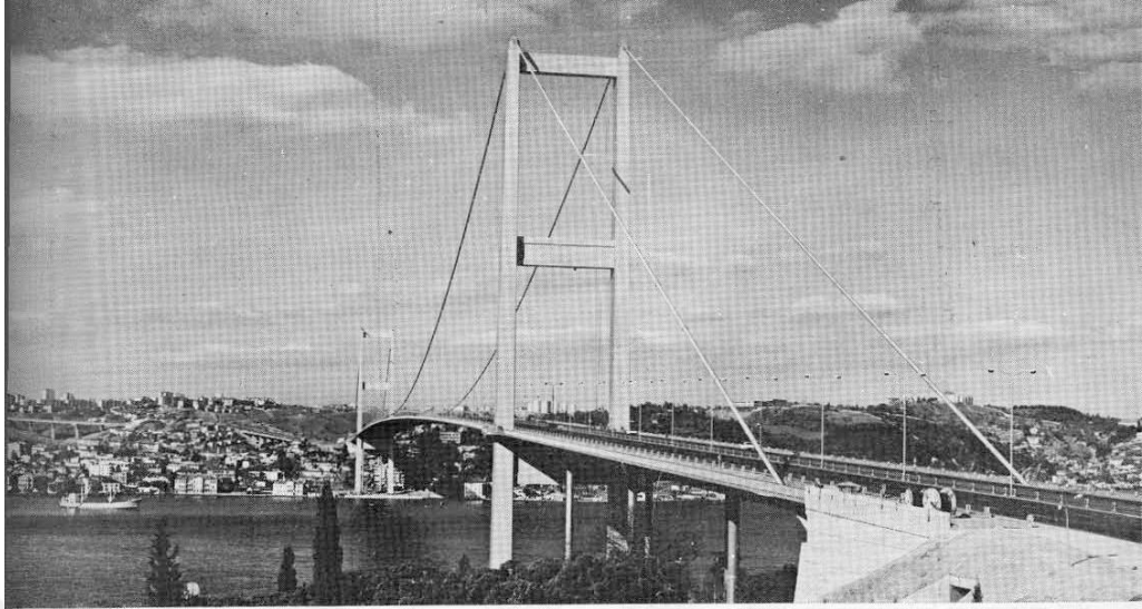
Figure 4.14 The View of the Bosphorus Bridge from Beylerbeyi in 1975. Arkitekt. "Boğaziçi Köprüsü", Vol.1975 No. 1975-01 (357), 7, 1975.
