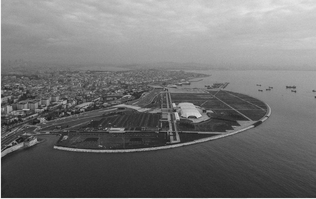
Figure 5.23 The Yenikapı Coastal Land Reclamation Project (Photo: Doğukan Bilgin). https://xxi.com.tr/i/tasarim-yonetiminde-sekulerlesme-sorunsali-kamusal-alanlar-ve-imamoglu
