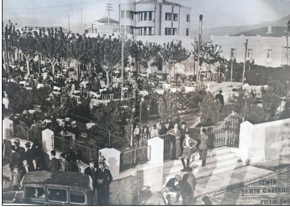
Figure 27. General view of Şehir Casino in early 1940s (Source: Kent Konak KNK Magazine , 2015)
