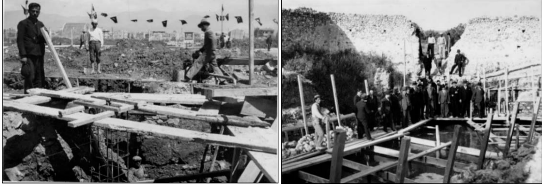
Figure 11. Photographs showing the construction of ICP, mostly done by the city's citizens. According to the interviewees, many master builders worked without payment to construct its surrounding walls, which were demolished in 1991 27 (Source: APIKAM Archive; IZFAS album )
