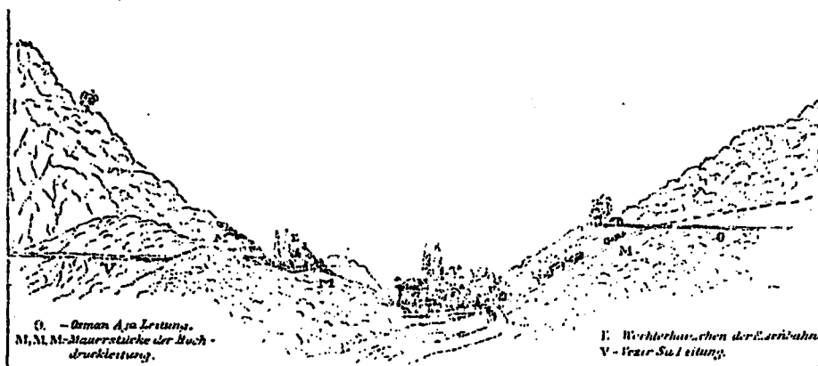
Figure 3.29:[Weber 1899/I; p.16] Northern view of the Melez valley, and the stone-pipe inverted siphon of the Karapınar system
