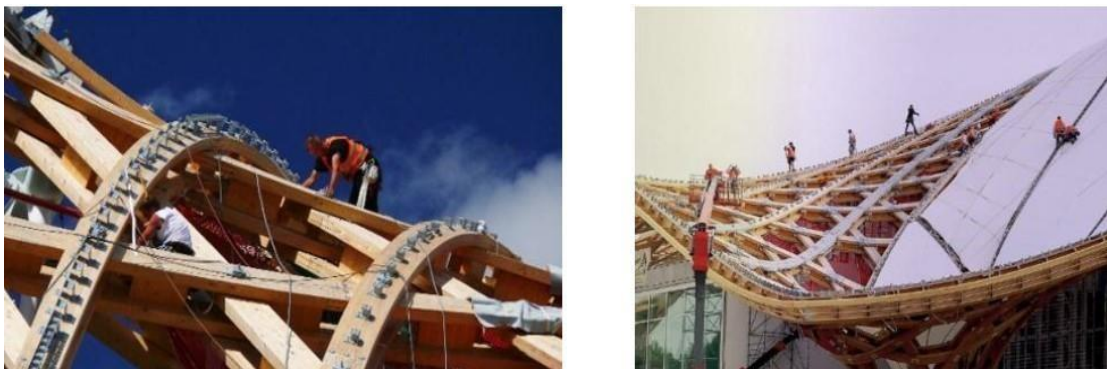
Figure 4.43 Wooden frame and roof system (Ban, 2010)
