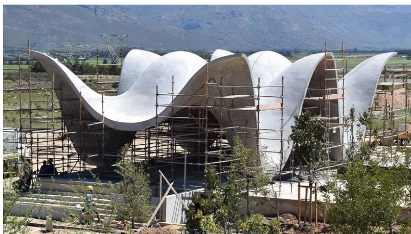
Figure 4.54 Bosjes Chapel under construction
