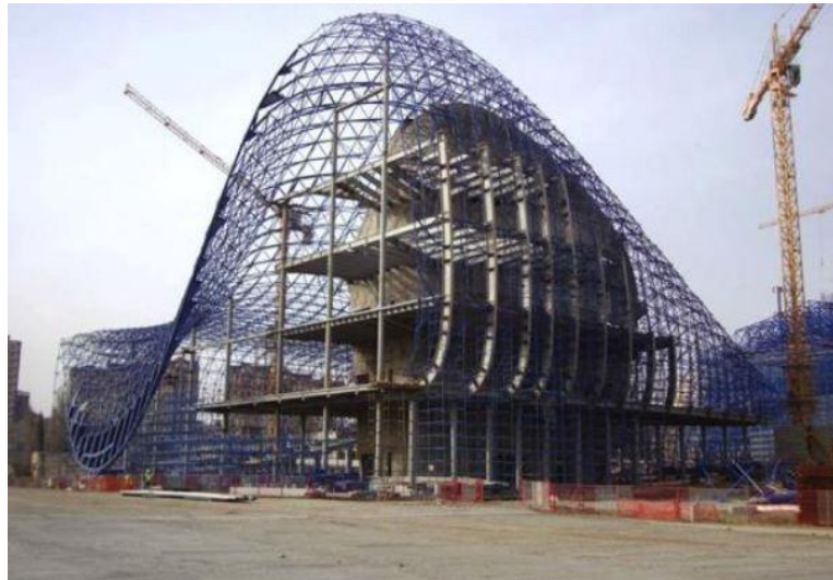
Figure 4.30 Space Frame and Core RC structure (Tarboush, 2019)
