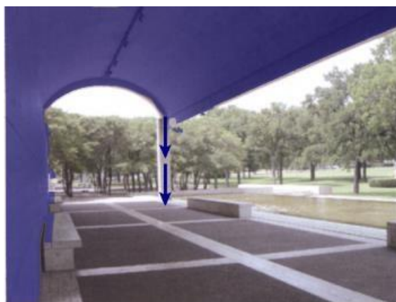
Figure 4.12 Membrane action and load path in the museum shell (Park et al, 2007)
