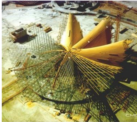
Figure 4.51 Temporary structure underneath the shell (CompetitionLine, 2012)
