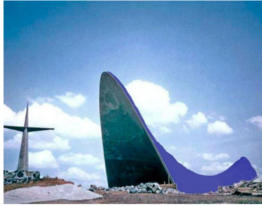
Figure 4.3 Shell under membrane action (Chris J.K Williams)
