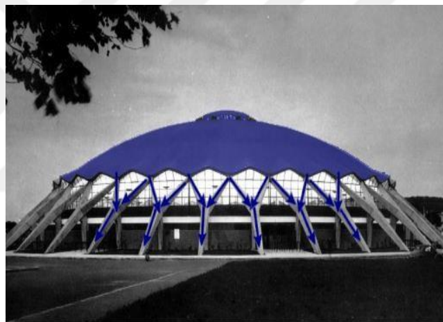
Figure 4.21 Membrane Action and the Load paths of the dome shell (New York: Praeger, 1963)
