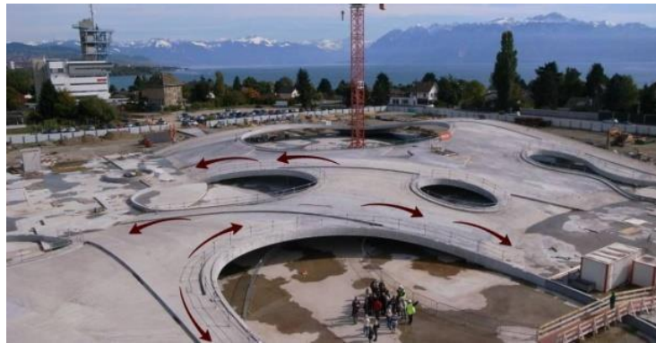
Figure 4.38 Load Path on the big shell (Weilandt 2009)
