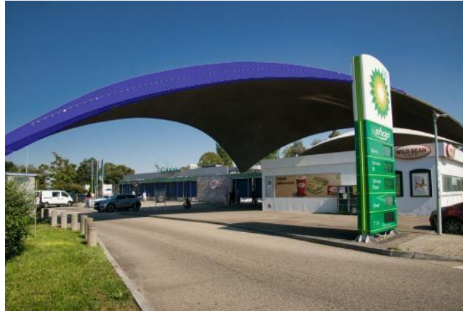
Figure 4.7 In Plane Membrane Forces in the Shell (Highlighted in Blue) (Nicolas Janberg)
