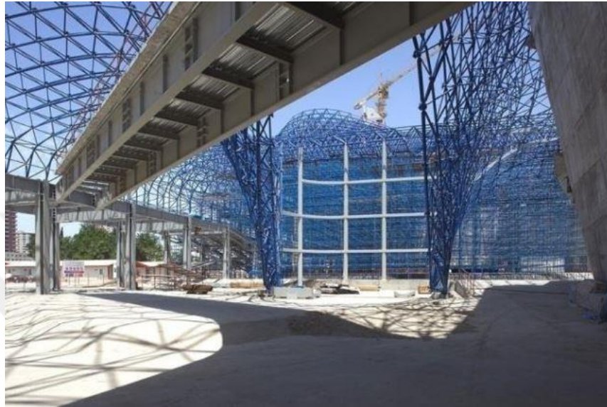
Figure 4.31 Steel bridge of Heydar Aliyev center (Tarboush, 2019)
