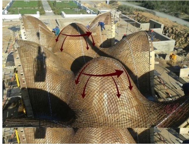
Figure 4.55 Load Path ( https://www.peri.co.za/projects/cultural-buildings/bosjes-chapel.html )
