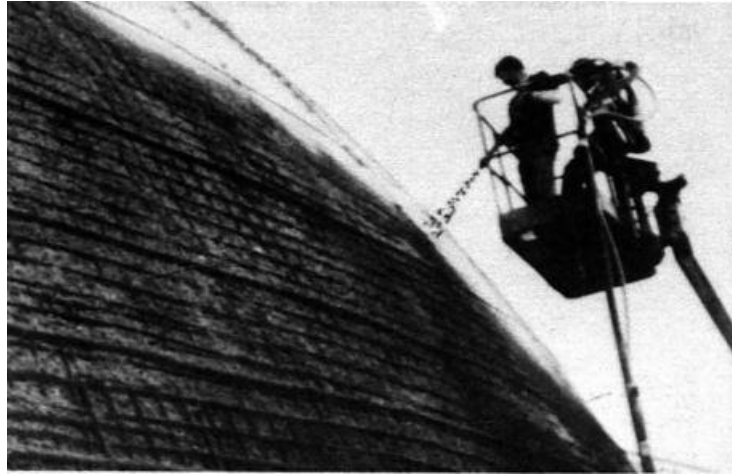
Figure 4.17 The first layer of concrete being shotcreted (Sobek,1987)
