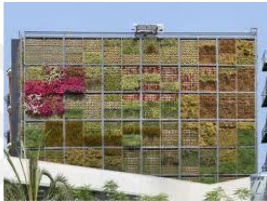
Figure 2.14 Six-storey tall green wall by architect Jose Maria Chofre, constructed with modular cubic containers, sandwiched between two metal grids.
