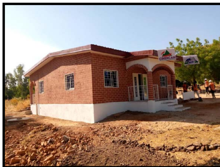
Figure 4.7: Earth-cement pilot project in Pitoa Source: 237infos (2021)
