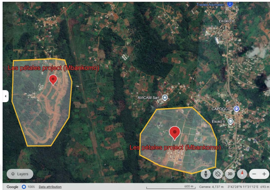
Figure 5.3: Aerial view Les Pétales project
