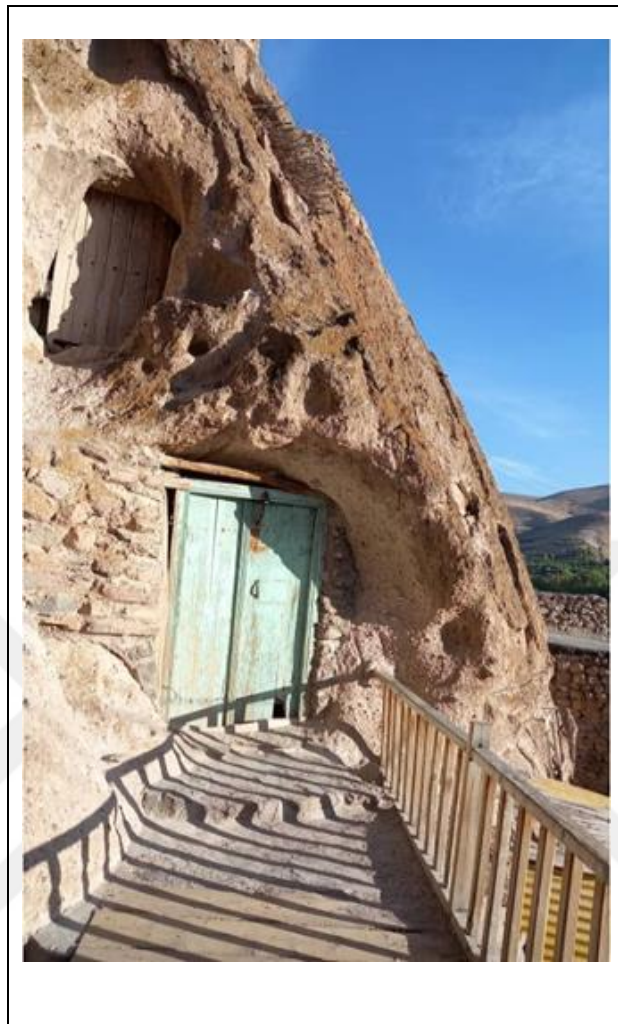
Figure 4.12. Example of entrance doors [15].
