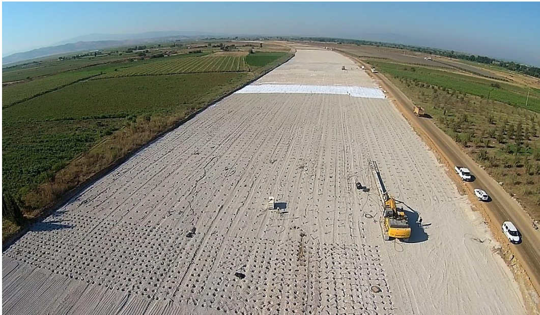
Figure 3.1. Prefabricated vertical drain installation in the Karacabey Plain
