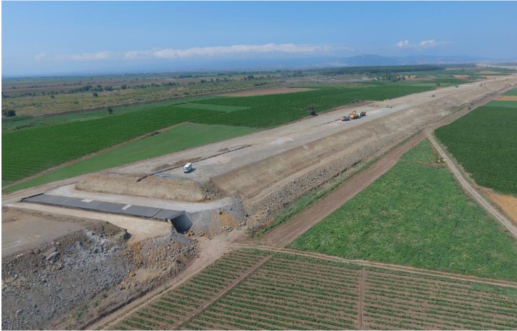
Figure 3.2. Embankment construction on the Karacabey Plain
