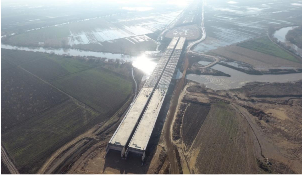
Figure 3.5. Flood plain view of Karacabey Plain
