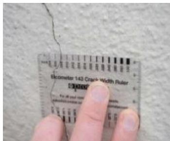
(a) Crack Width Measuring
