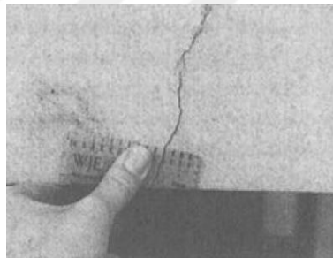
Figure 2.1. Manual Crack Measurement Using a Width Gauge (Farmer, 2004)
