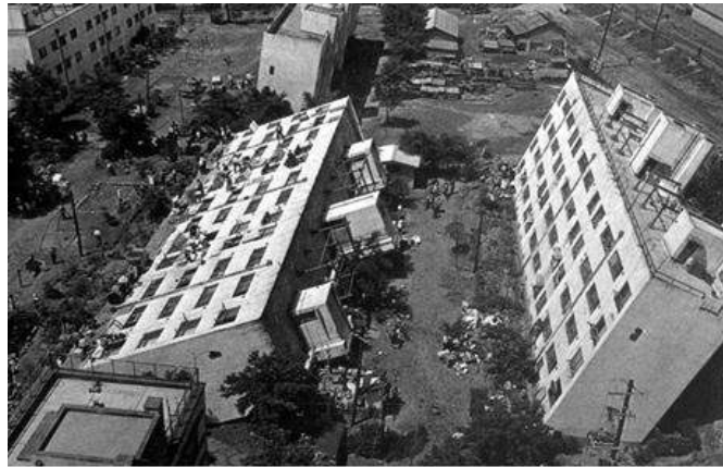
Şekil 2.11. Niigata Depremi 1964 (University of California, Steinbrugge Collection)
