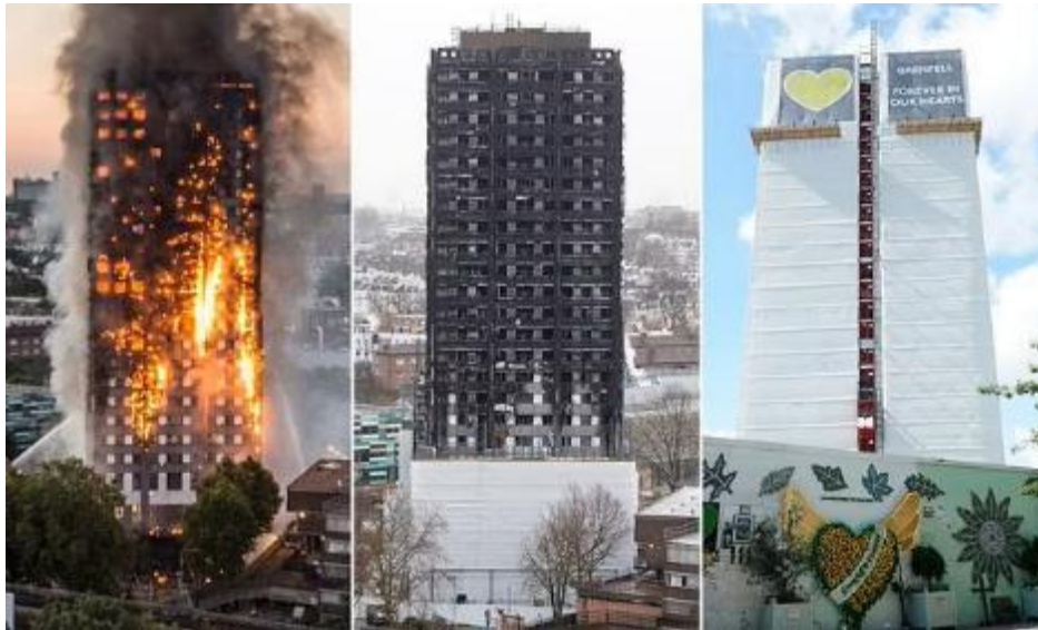
Figure 3. Grenfell Tower façade during post-fire inspection (Dan Woodland, 2024)
