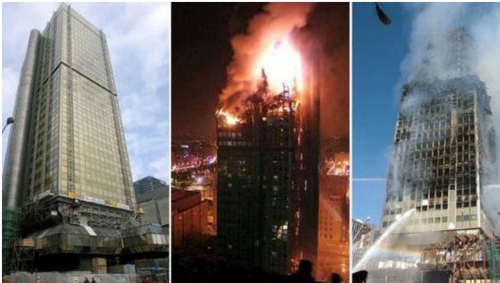
Figure 2. Windsor building fire (2005) (Luminex Inc, 2024)
