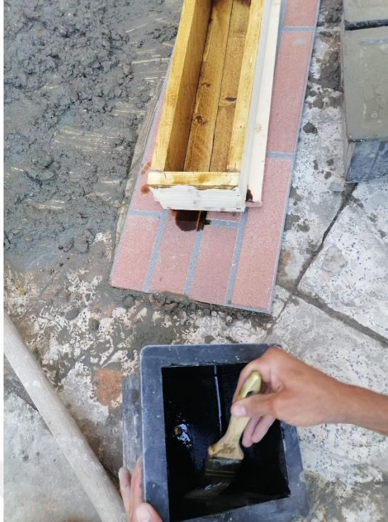
Figure 3.6: Oiling The Molds.
