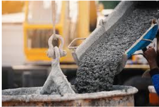
Figure 2.2: Self-Compacting Concrete Production.
