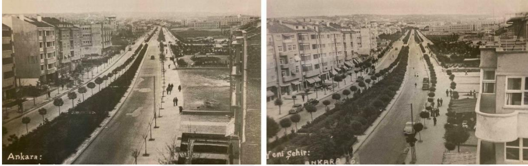
Figure 3.32 Both photographs of Atatürk Boulevard taken from about the same point to the south are from the late 1940s. It is possible to see that the construction on the boulevard has increased, and cafes and shops on the ground floors have opened in the short time that elapsed between the dates of the two photographs. In the photograph on the right, Özen Lokantası is on the west side of the boulevard (Right side on the photograph).
