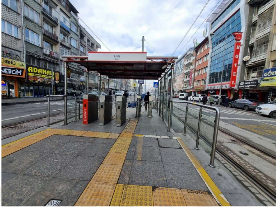
Figure 5.22 Photo of Düvenönü Tram Station entrance
