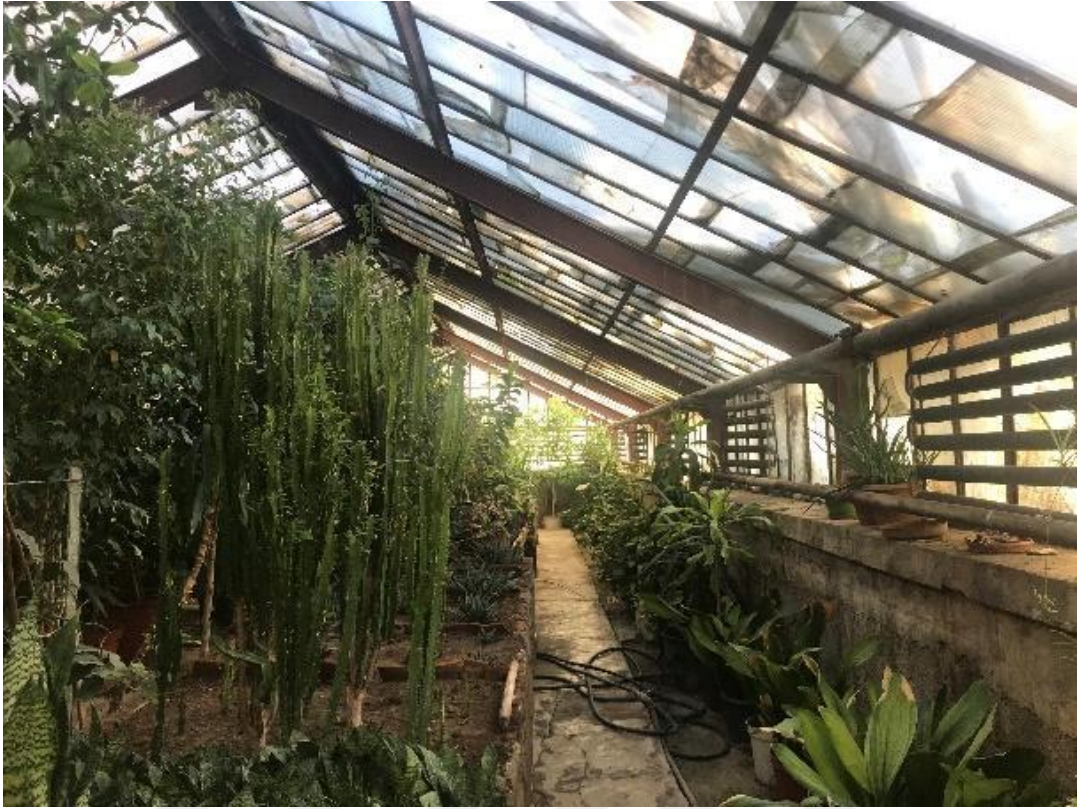
Figure 6.2 A greenhouse in sugar factory campus (Öztürk, 2019).
