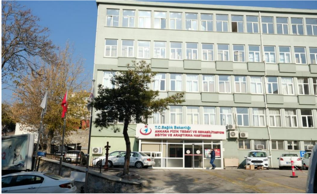
Figure 3.18. Ankara (Altındağ) Physical Medicine and Rehabilitation Education and Research Hospital, Ankara (photograph by I. Şenses, February 2021)
