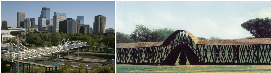
Şekil 2.28 : Siah Armajani’nin Irene Hixon Whitney Bridge ve Bridge Over a Tree.( http://artasiapacific.com , Url- 30)
