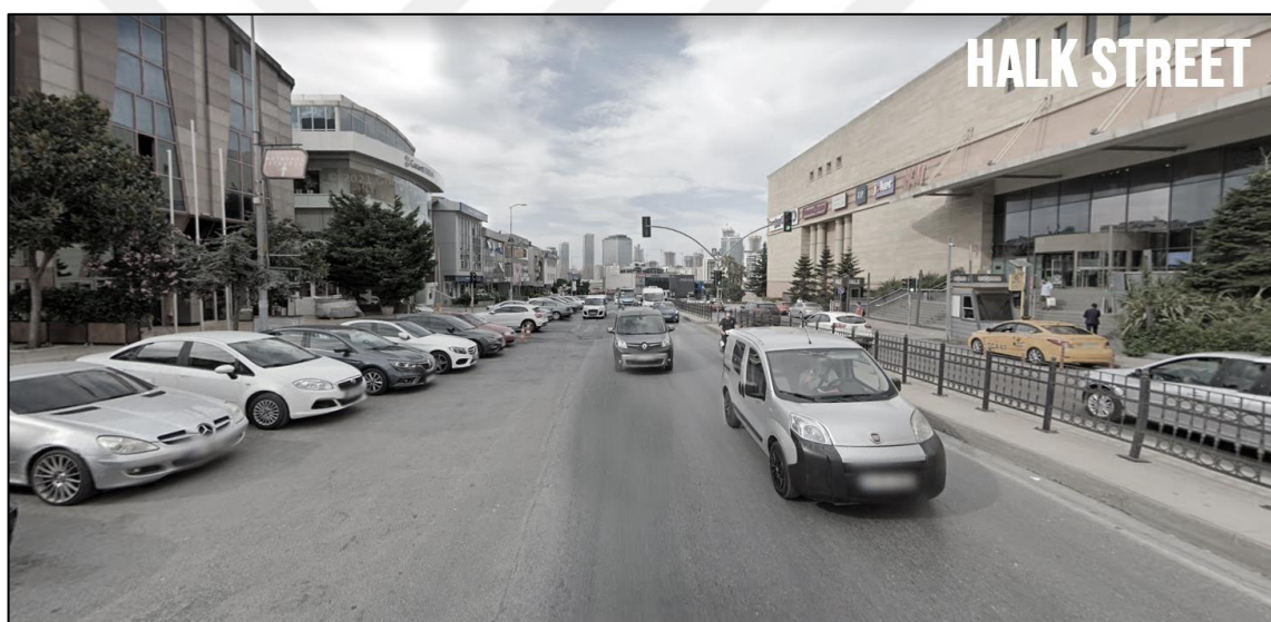
Figure 6.45 Halk street, which is the eastern border of the area [202].
