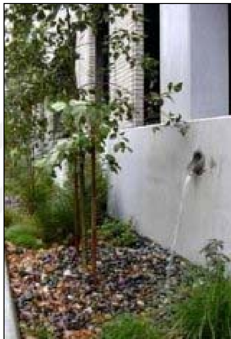
Figure 2.17. Downspout disconnect application [77]
