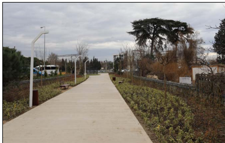
Figure 3.18. Tuzla Valley of Life lighting equipment [98].
