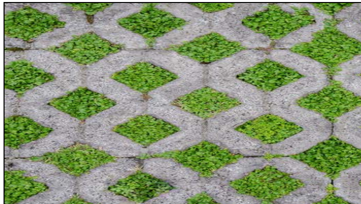
Figure 2.21. Permeable pavement application [55]
