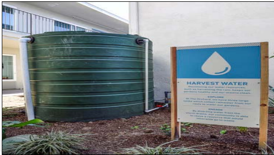
Figure 2.18. Rainwater collection system [55]
