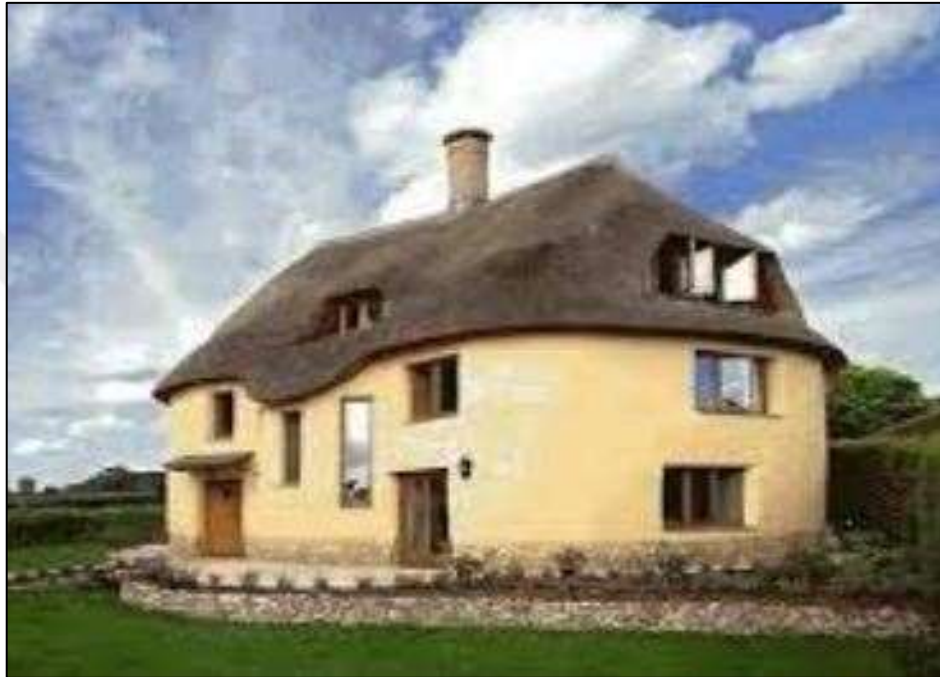
Figure 4.8: Example of Using Cob in Contemporary Architecture.
