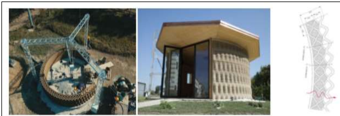
Figure 2.16: 3D- Printing Technique in Gaia Project (WASP, 2018).
