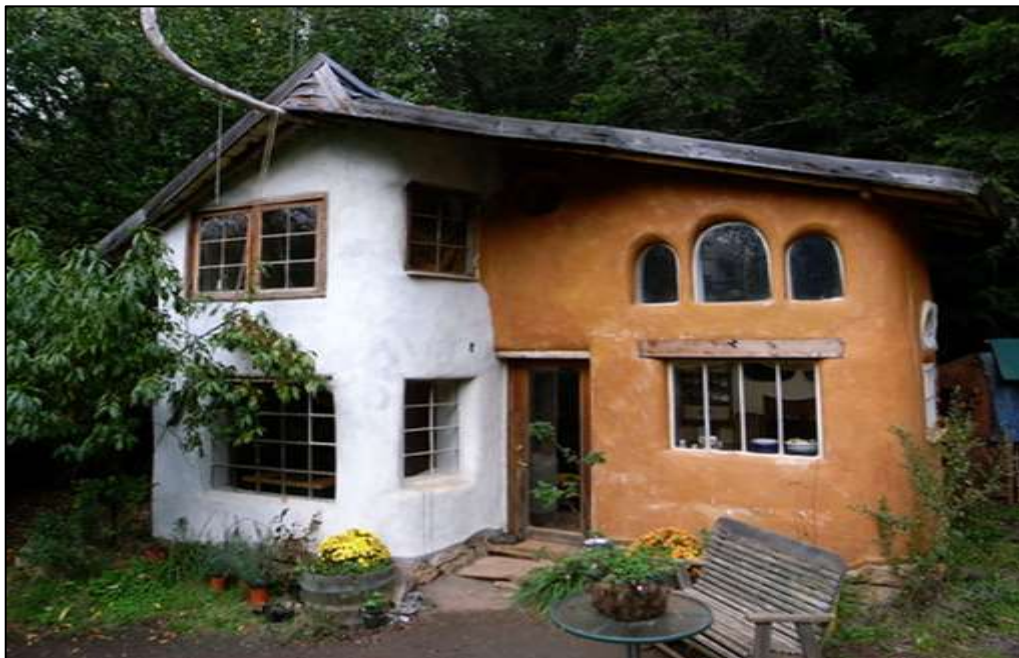
Figure 2.28: Fusion Between the Past and the Present.
