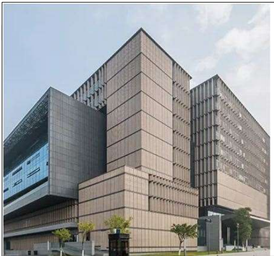
Figure 4.7: Using Example of Structure Adopted Terracotta in the Facades.
