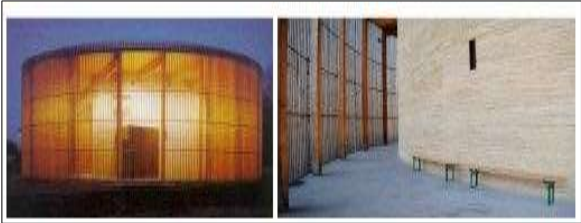
Figure 4.5: Building Chapel of Reconciliation.
