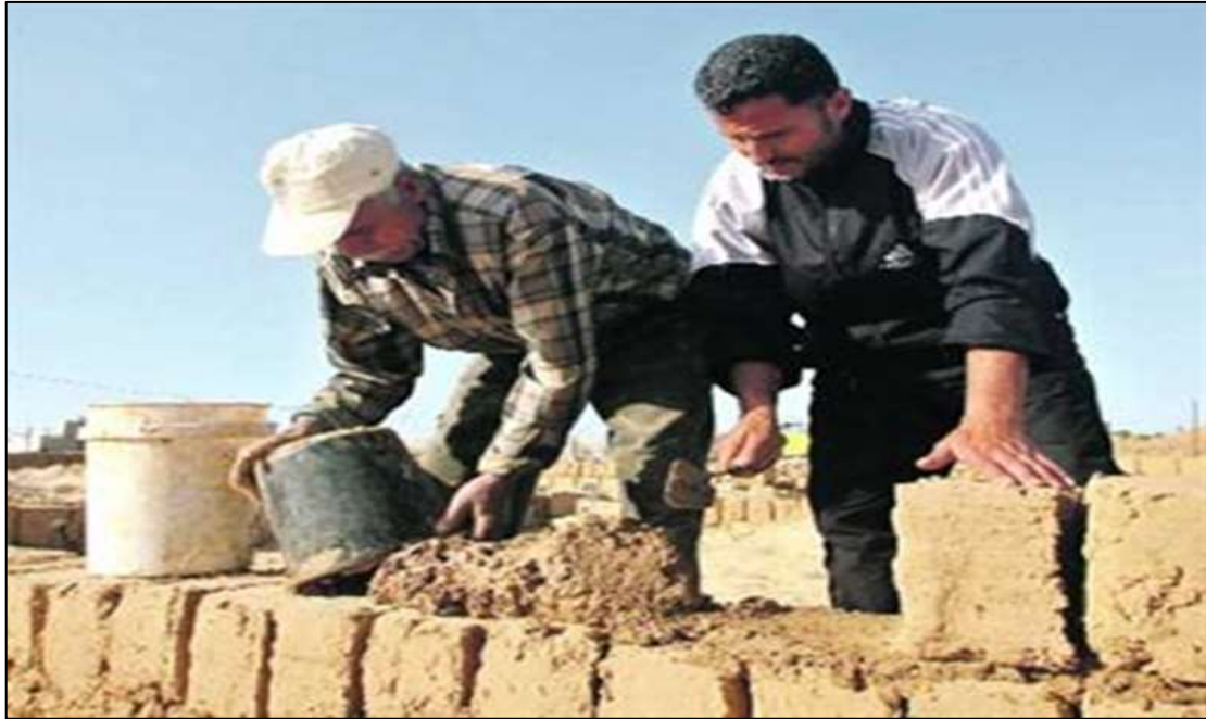
Figure 2.5: Reinforcing the Walls with Mud.
