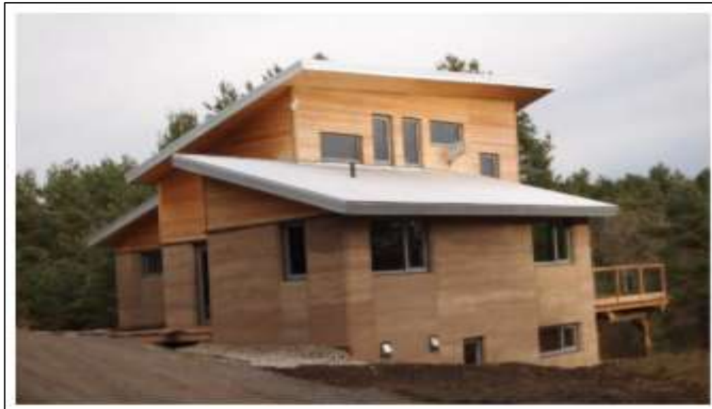
Figure 2.15: Rammed Earth Home Djamil (2016).
