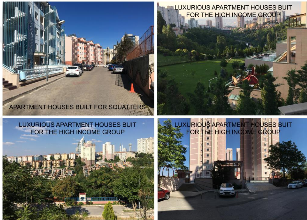
Figure 12- The apartment houses constructed for the former gecekondu dwellers and higher income groups in the first three phases of Dikmen Valley Urban Transformation Project (source: author).
