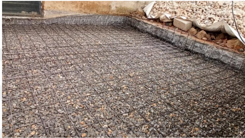
Figure 4.4 Steel mesh and aggregate laying process
