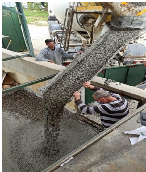
Figure 4.5 Ready-mixed concrete pouring process
