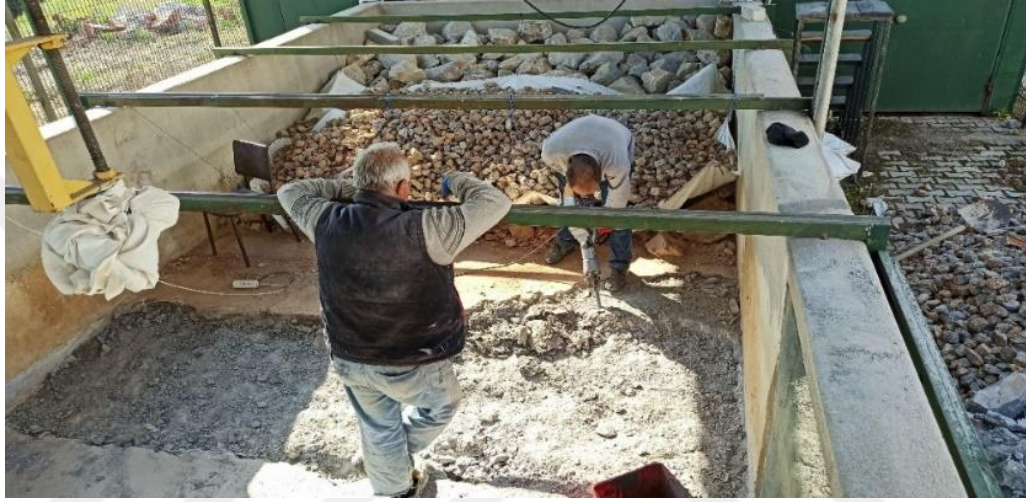
Figure 4.2 Breaking the ground to widen the sandpit
