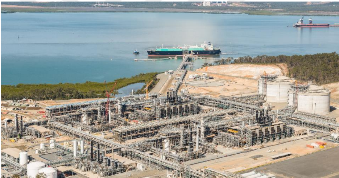
Figure 11: Gladstone LNG Terminal, Australia
