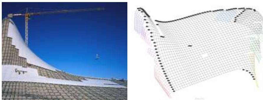
Figure 2.27: Construction of Haydar Aliyev Centre's panels, Zaha Hadid Partners, 2013 ( https://www.rok-office.com/projects/1000-haider-aliyev-cultural-centre/ )
