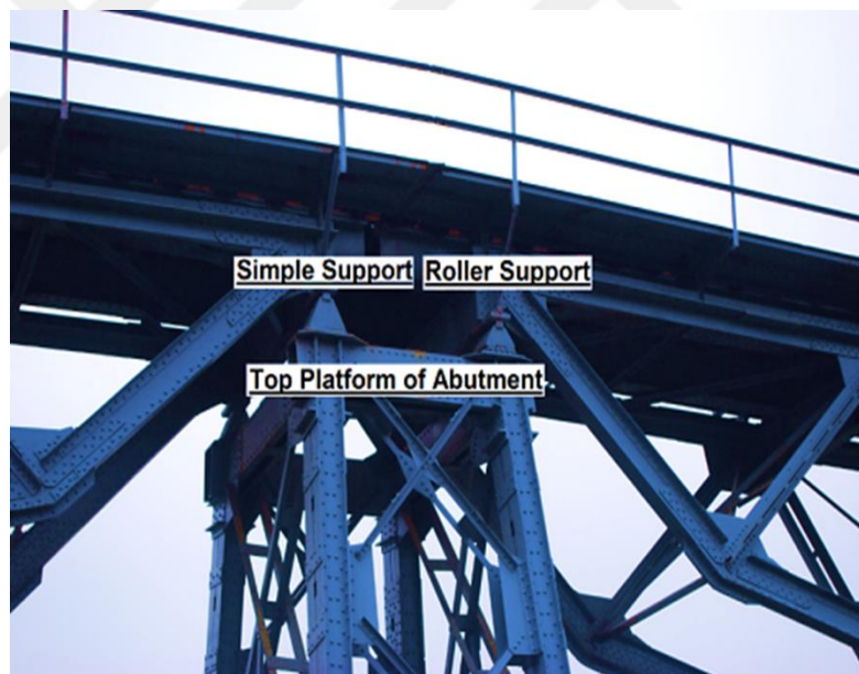
Figure 5.20 Actual column to support detail (Personal archive, 2015)
