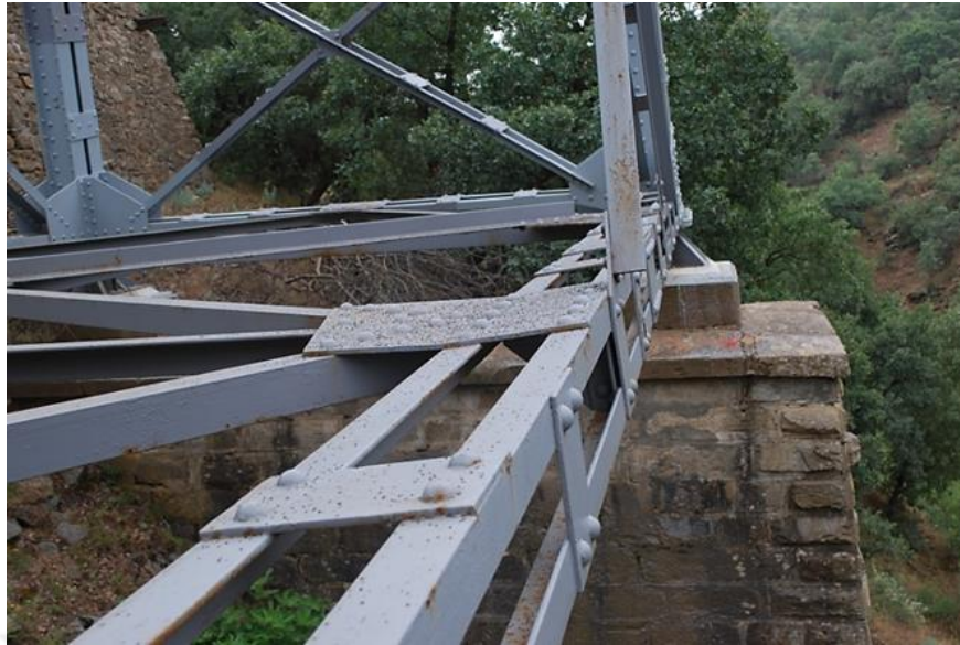
Figure 5.12 Horizontal bracing (Personal archive, 2015)
