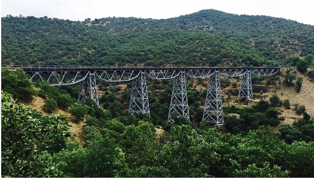
Figure 3.2 The current picture of the 199 + 325 railroad steel bridge (Personal archive, 2015)
