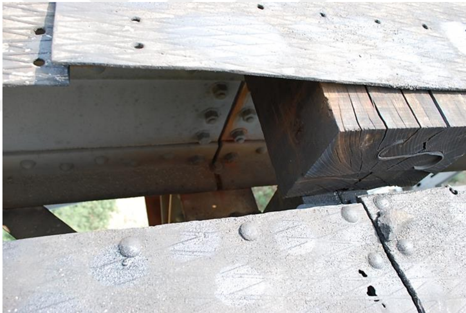
Figure 5.7 Sleeper on stringer (Personal archive, 2015)
