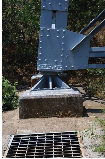
Figure 5.10 Masonry base support (Personal archive, 2015)
