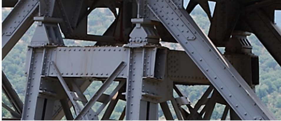
Figure 5.14 Top frame of abutment (Personal archive, 2015)
