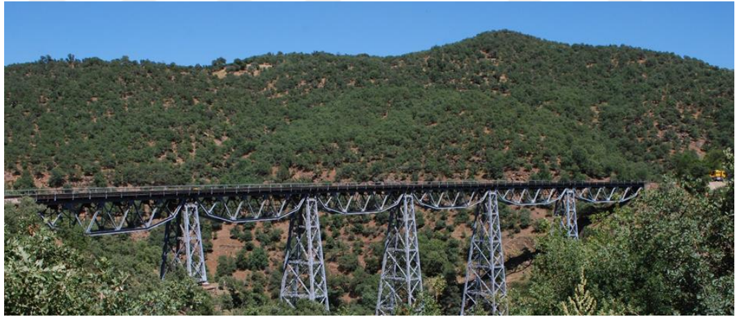
Figure 1.1 199+325 Steel railroad bridge (Personal archive, 2015)
