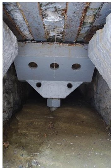
Figure 5.9 Anchored rod (Personal archive, 2015)
