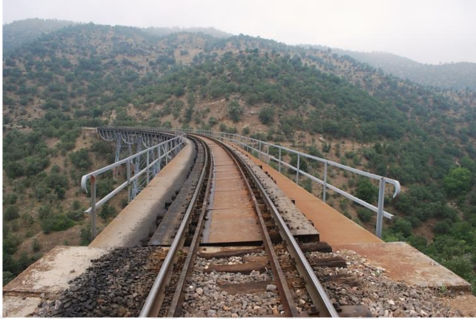
Figure 5.6 Rails, footpath and railing (Personal archive, 2015)
