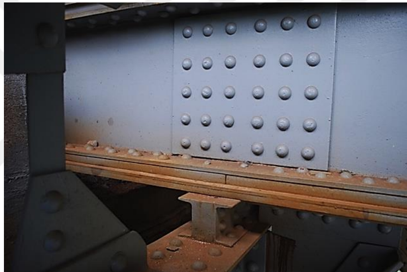
Figure 5.5 Detail of the stringer (Personal archive, 2015)
