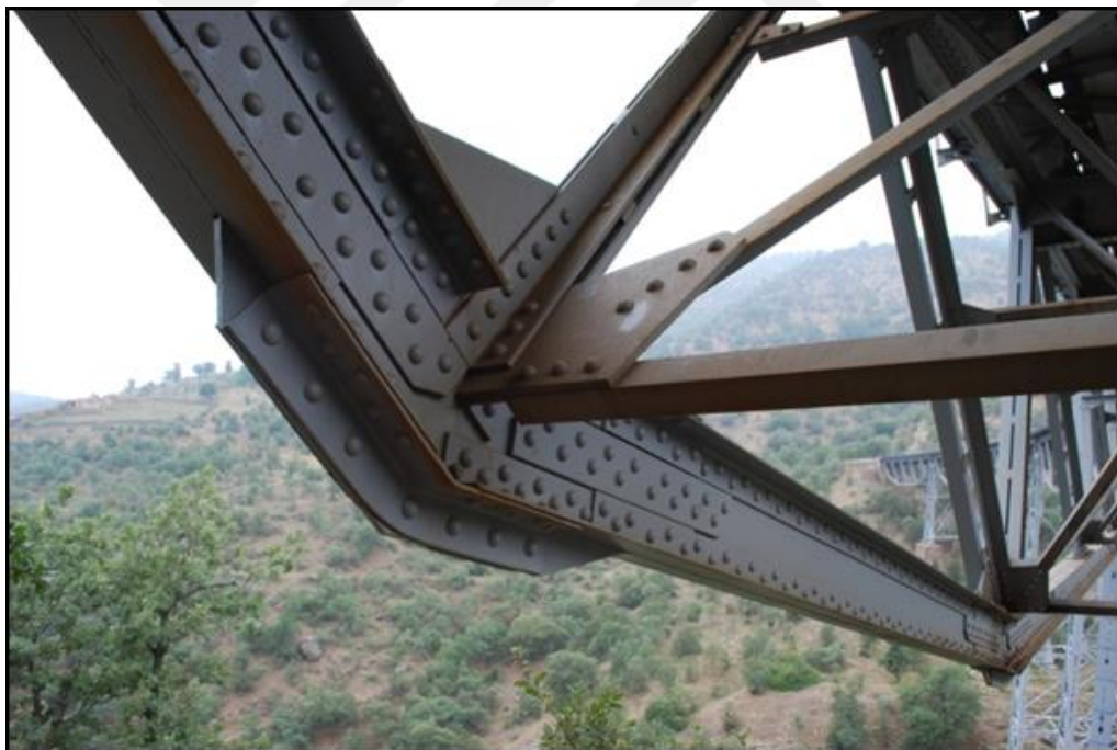
Figure 5.3 Strengthened joint detail (Personal archive, 2015)
