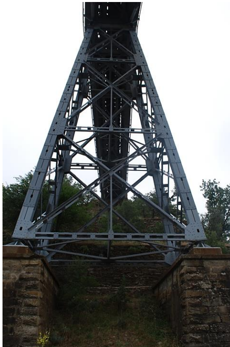
Figure 5.11 Abutment (Personal archive, 2015)
