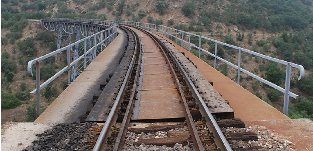
Figure 3.4 The platform view of 199+325 steel railroad bridge (Personal archive, 2015)
