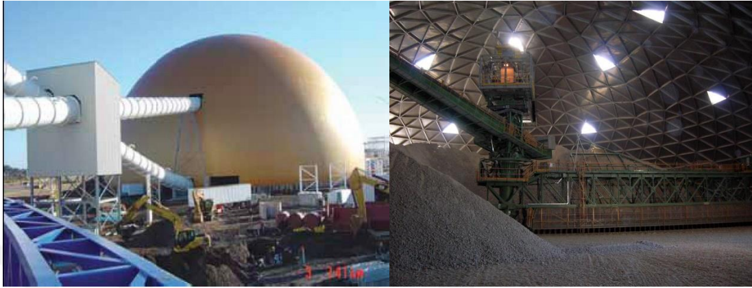
Figure 6: Dome Closed Storage Examples
