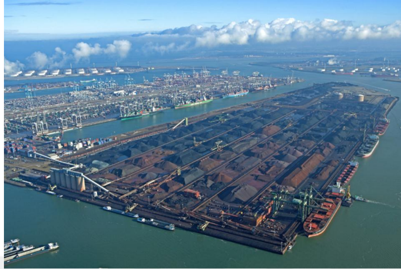
Figure 3: General View of Dry Bulk Terminal Layout
