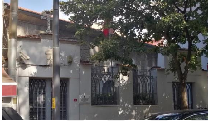
Figure 28: The Exterior of Agios Georgios Greek Orthodox Church [85].
